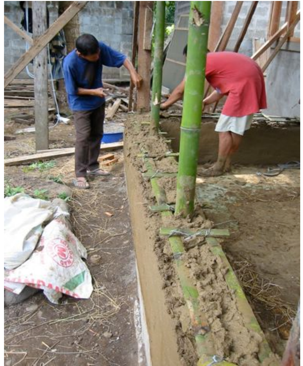
In Gingoog - 300 mm thick walls
